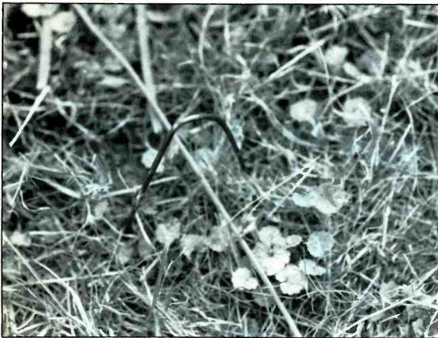
Fig. 4 Use of coat hanger ends to hold down radials. Push ends down into ground firmly.
