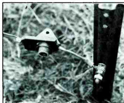
Fig. 3 Dipole-to-coax connector. Its ground side connects to ground stake.
